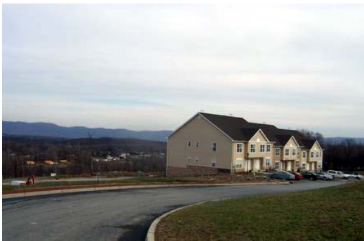
Newer development resulting in interrupted viewshed
