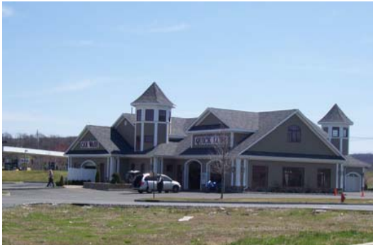
Despite being poorly landscaped and setback from the road, the design (in terms of form and materials) of this auto-oriented use building (a car wash) responds well to local aesthetic character
