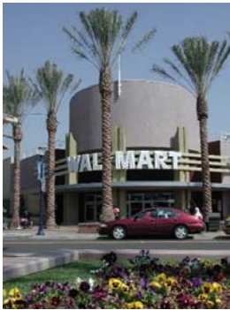
Three examples showing that “big-box” stores can be held to higher design standards. These examples, in varying degrees, are more pedestrian friendly, better landscaped and more aesthetically pleasing than the typical large-scale retail configurations observed throughout the country
