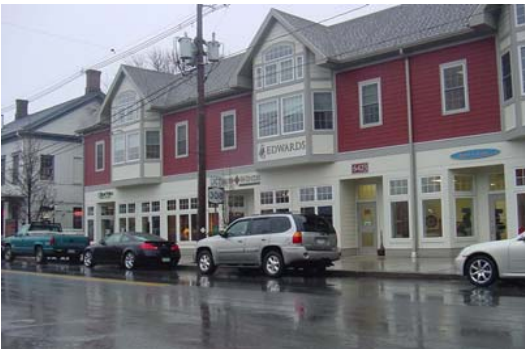
A good example of a pedestrian friendly, mixed-use hamlet district streetscape in the Town of Newburgh with stores on the ground level and residential/offices above
