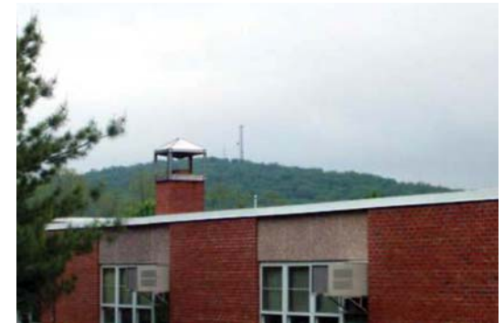
A communications tower in the Town of Newburgh located on top of a ridge line (undesirable)
