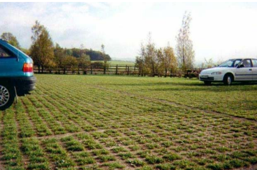
Porous block pavers offer can be an environmentally sensitive and attractive driveway treatment
