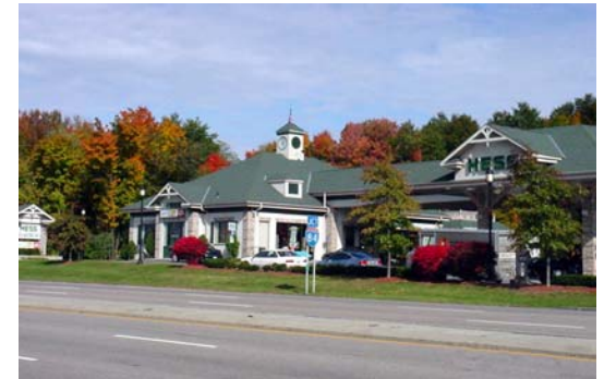
This Hess gas station located at the intersection of I-84 and Route 9 in Dutchess County is an example of a national chain incorporating locally responsive design elements into its building (desirable)
